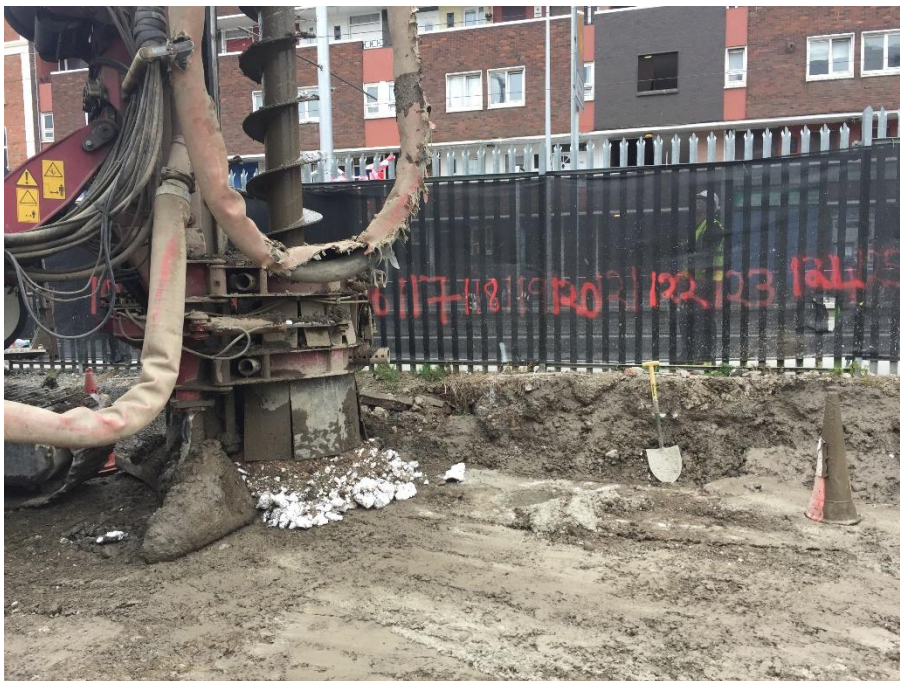
Secant Piling Works Progressing along Dominick St. Lower Elevation
